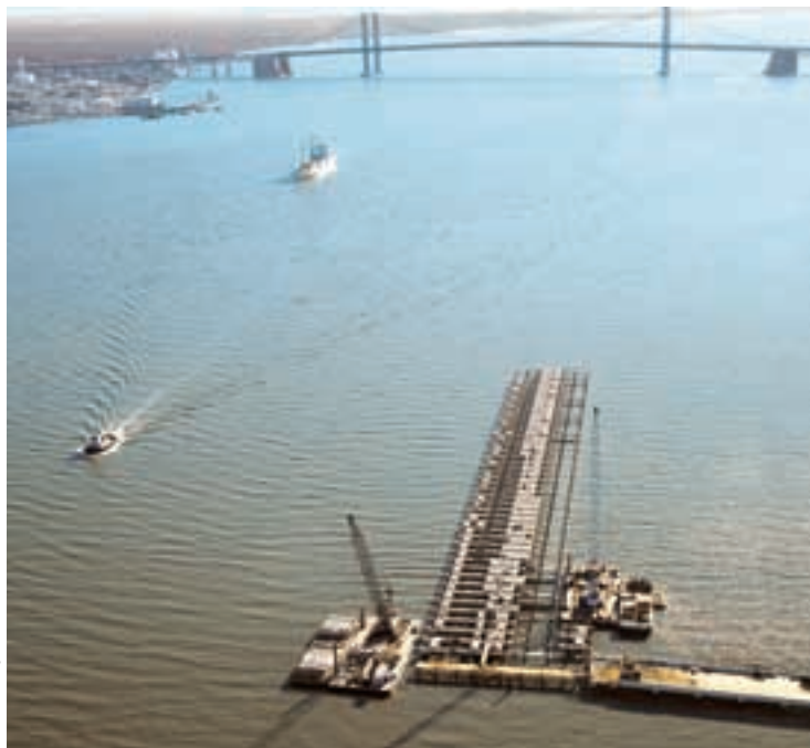
The Port of Wilmington’s dedicated auto carrier berth project is progressing on schedule with the completion of the trestle and the placement of the pile caps at the berth.
