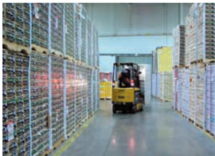
The Port of Wilmington owns and operates the nation's largest dockside cold storage warehouse facility encompassing 700,000 square feet. Shown is Chilean fruit stored at the Port's newest cold storage warehouse E which includes 16,000 square feet of controlled atmosphere rooms.
